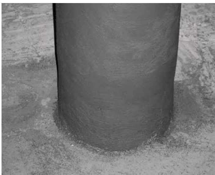
Above: Support column repair from beginning to end, using the Metallock process.
